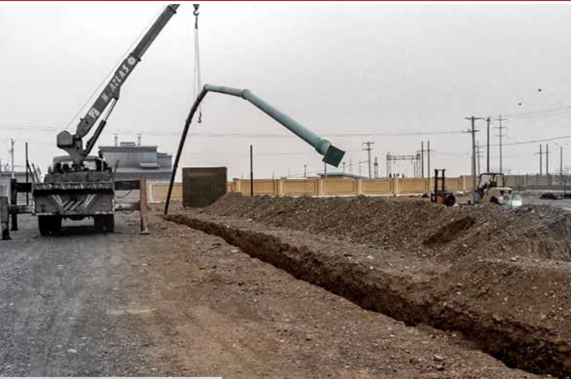
DN150 Q.R flex pipe deflection during the installation
